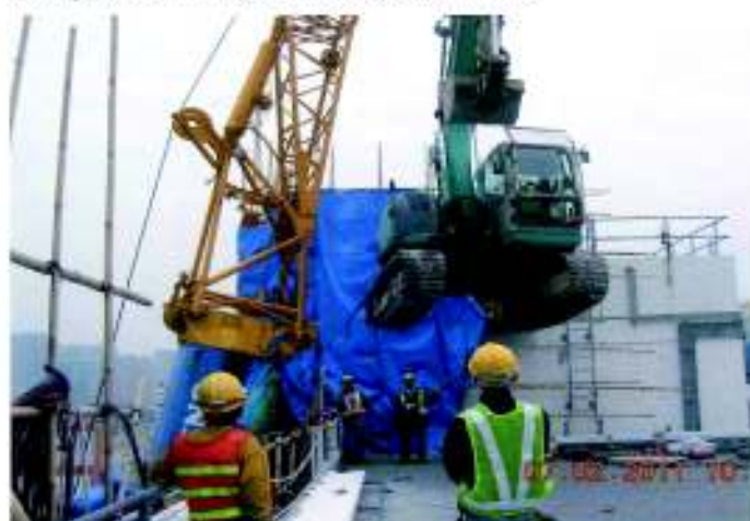
Lifting of mechanical plant by mobile crane
