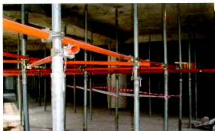
Props with horizontal tubular bracing by couplers
