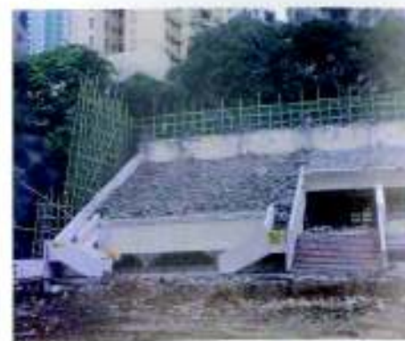
9. Demolition of end bay completed
