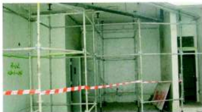
Frame system used as propping for excessive floor height
