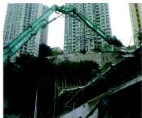
4. Crashing front portion of main cantilever girder
