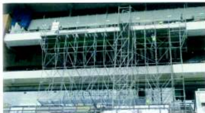
Frame system with platform at top for cantilever demolition
