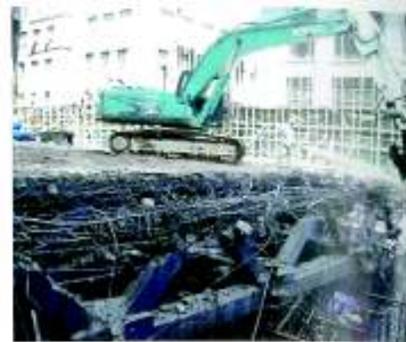
3. Crushing of top chord continues and removing rebars.
