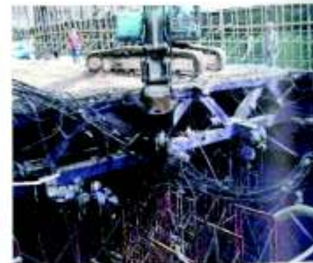
9. Removing rebars after completion of crushing
