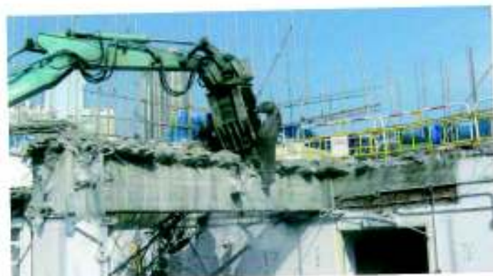
1. Crushing from mid span
