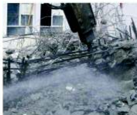
8. Breaking up remaining concrete
