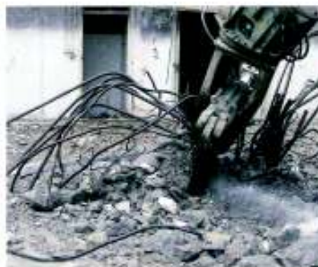
8. Crushing remaining concrete
