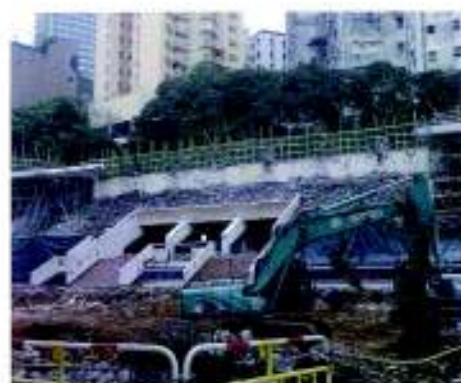
7. Crushing internal bays completed
