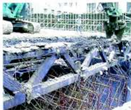
2. Crushing top chord of truss (props remaining in mid-span)
