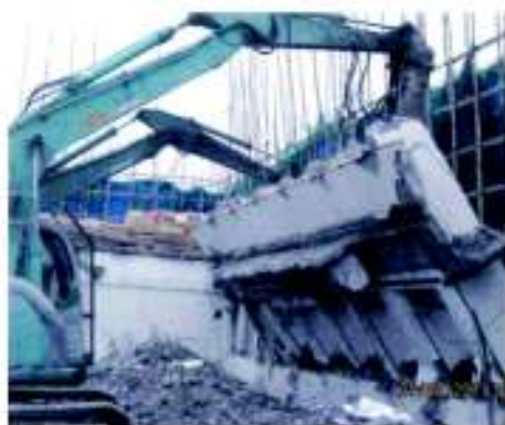
13. Pulling, wall coming down slowly with column rebar yielding
