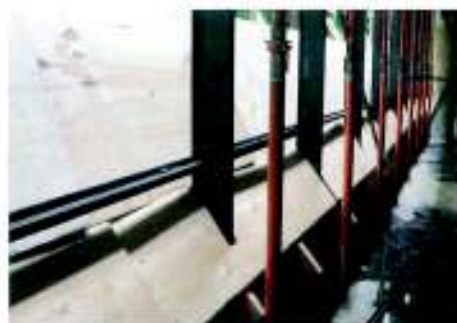
Example 5 Timber Catch Fans Installed between Scaffolding and Face of Building at Every Three Floors
