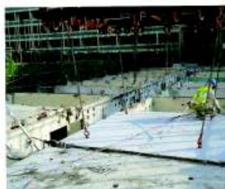
4. Securing Precast Slab Panel to Lifting Frame
