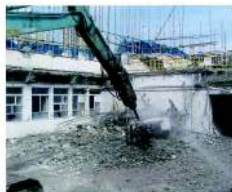
7. Column falls down slowly with rebars bending
