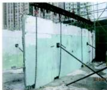
10. Securing Precast Wall Panel to Lifting Frame
