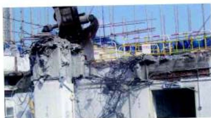
7. Crushing continues to other side of beam
