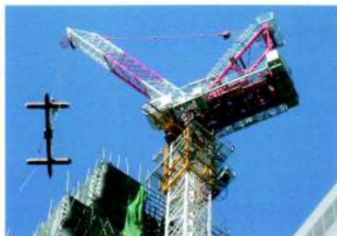
Lifting of demolished element by tower crane
