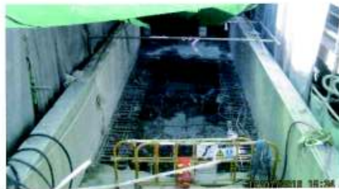
Debris from demolition being collected by platform
