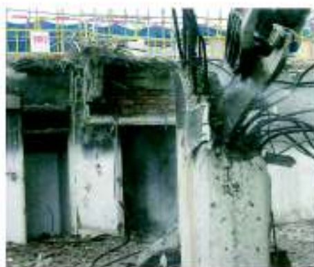
2. Crushing continues with water spraying
