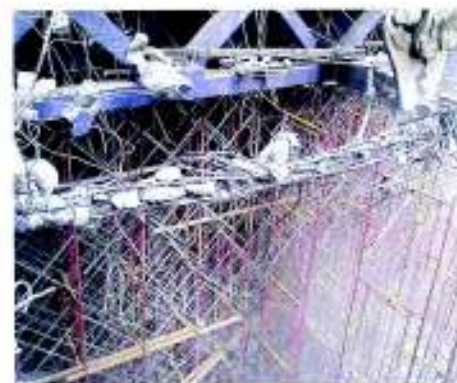
8. Crushing of bottom chords continues
