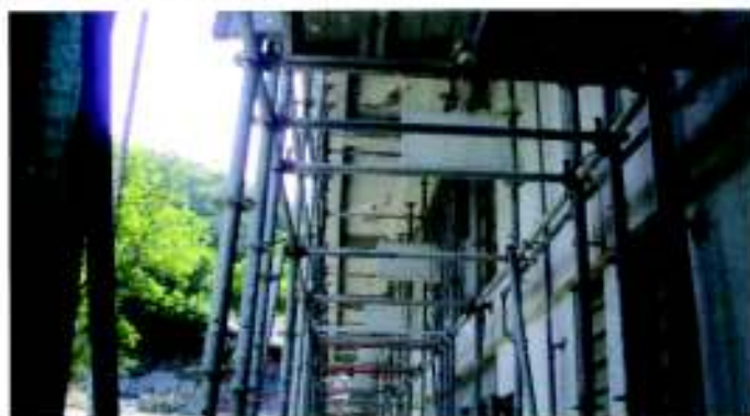
Platform integrated with frame system under cantilever
