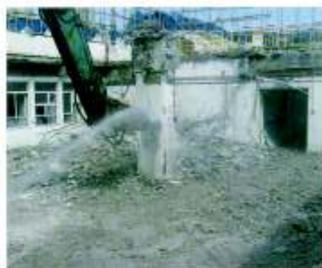
1. Breaking starts with area vacated
