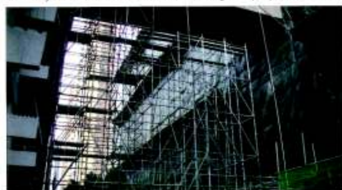
Propping using tubular frame system for demolition of overhead structure
