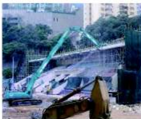
5. Crushing internal slab panels and secondary beams
