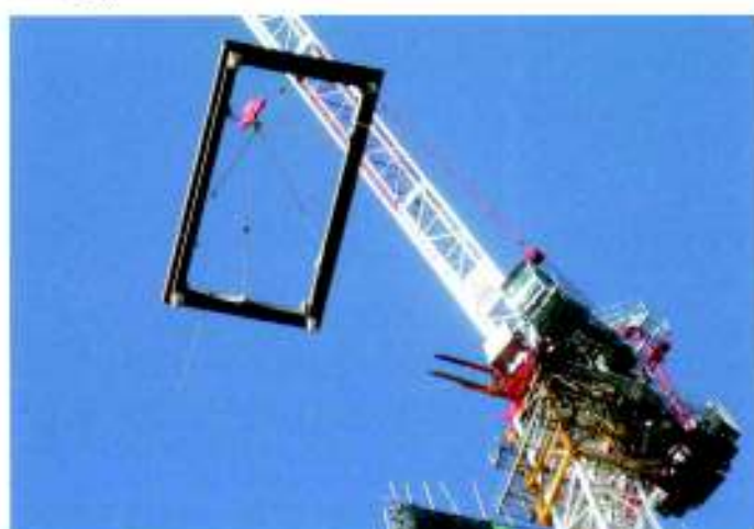
Lifting of demolished element by tower crane
