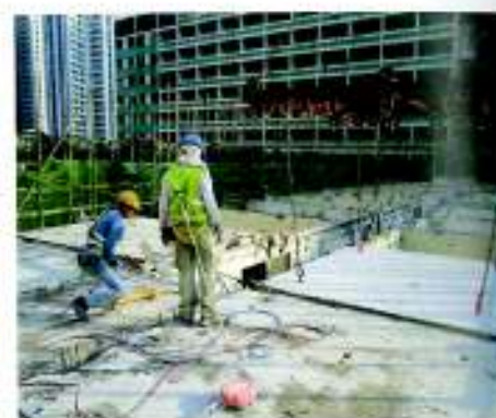
6. Jacking up Precast Slab Panel
