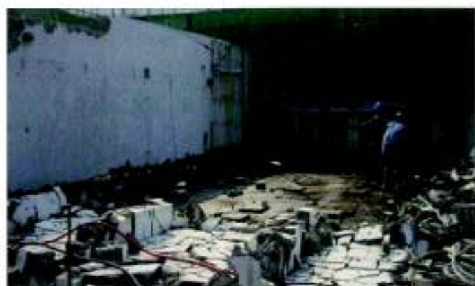
Example 6 Wall Demolition by Manual Method Using Chain and Block
