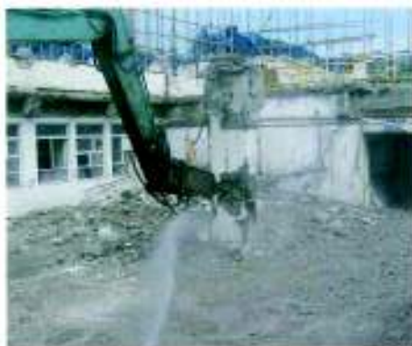
2. Breaking continues with water spraying
