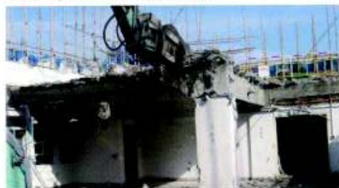
3. Crushing continues on right side of beam
