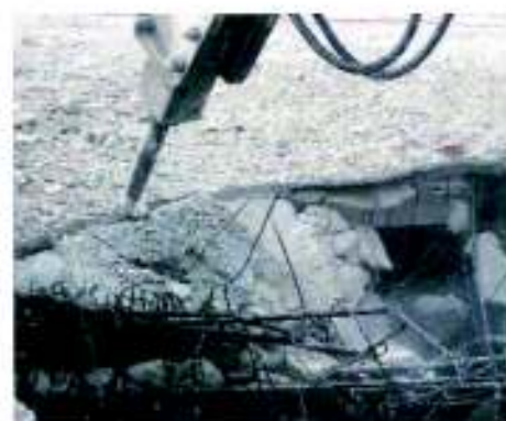
7. Breaking of slab continues
