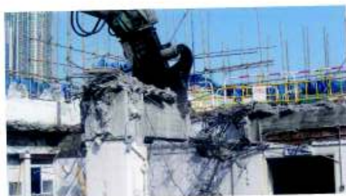
5. Crushing continues to other side of beam
