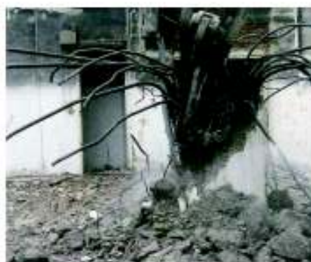
5. Splitting column concrete
