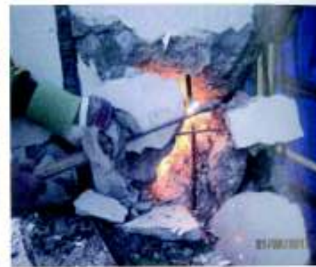
6. Cutting outer layer of rebar of column
