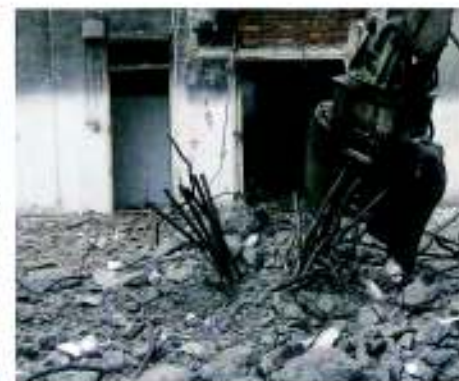
9. Cutting remaining rebar and finishing operation
