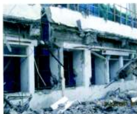
1. Breaking the upper wall / beam
