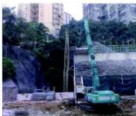
8. Demolishing end bay after removal of props
