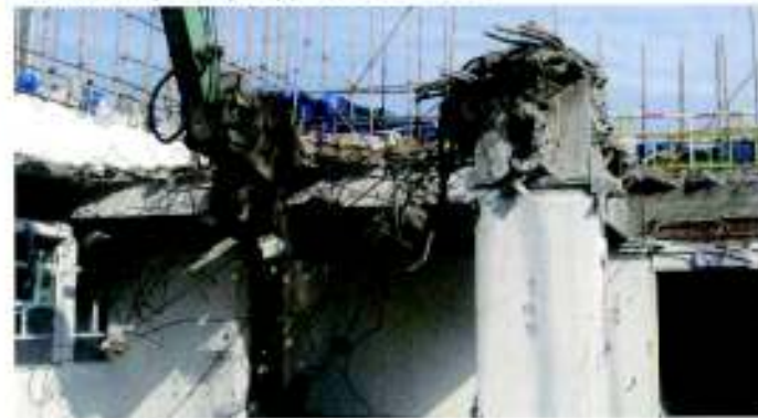
6. Crushing internal secondary beam
