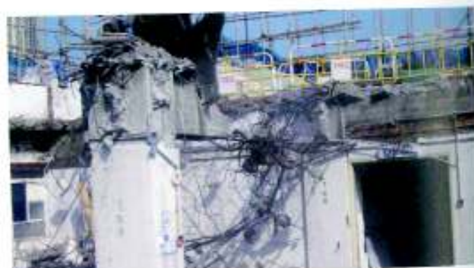
6. Crushing continues to other side of beam
