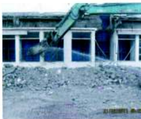
2. Breaking the lower fin / column
