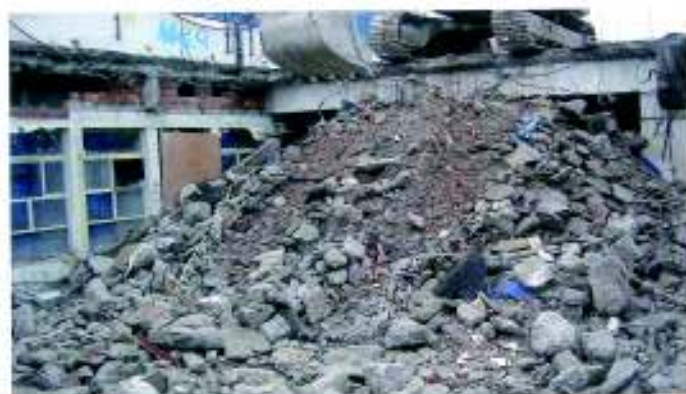
1. Ramp formed by concrete debris
