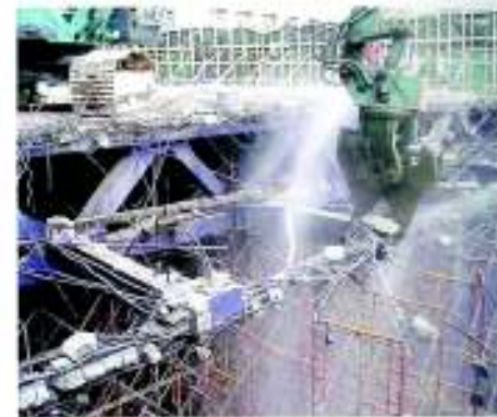
6. Crushing of bottom chords continues
