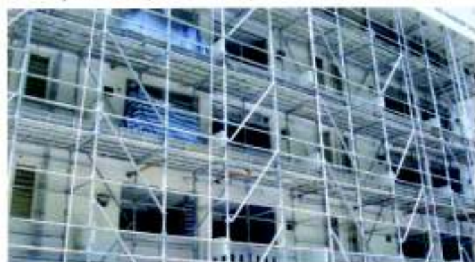
Frame system used as external scaffolding and prop to cantilever
