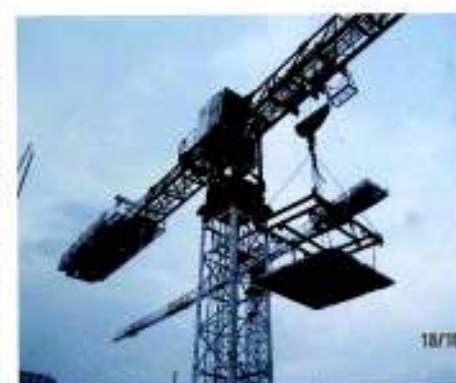
8. Lifting up Precast Slab Panel (2)
