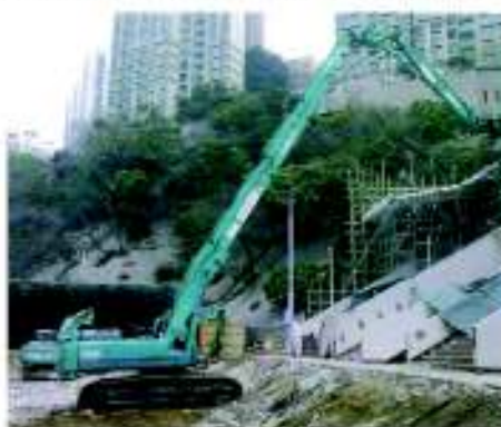
2. Crashing internal secondary beam
