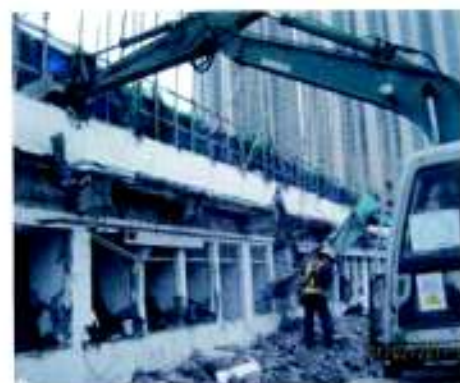
4. One holding the wall with the other breaking
