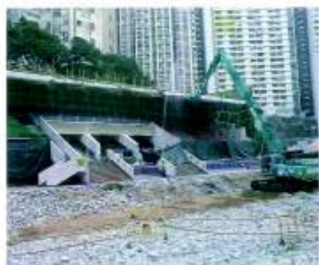
1. Crushing slab panels bay by bay
