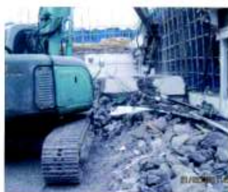
15. Breaking the concrete afterwards on ground
