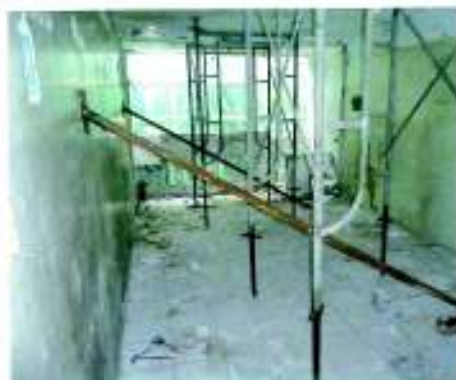
2. Installing Steel Props and Bracings
