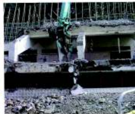
14. Clearing debris after seating demolition
