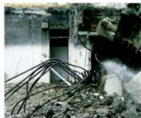
6. Crushing concrete off at bottom
