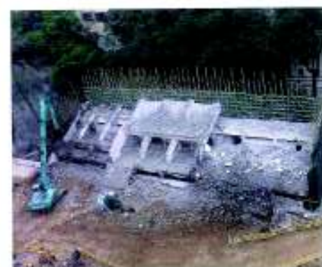
13. Demolishing spectator seating
