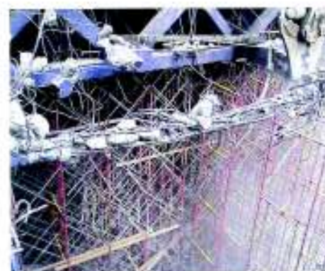
7. Crushing of bottom chords continues
