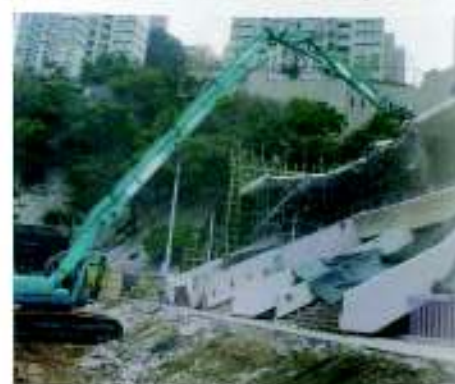
3. Crashing internal slab panel
