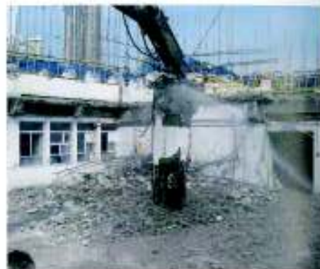
6. Pushing down column
