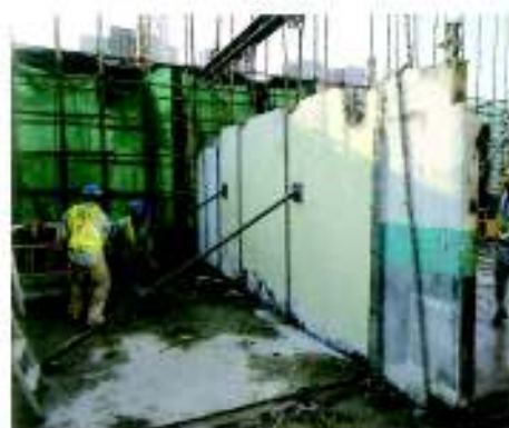
13. Jacking up Precast Wall Panel
