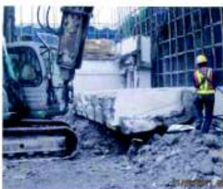
14. Cutting the inner rebar
