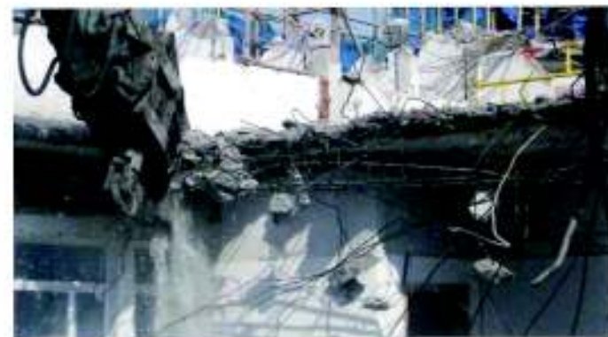
8. Finishing slab panel demolition
