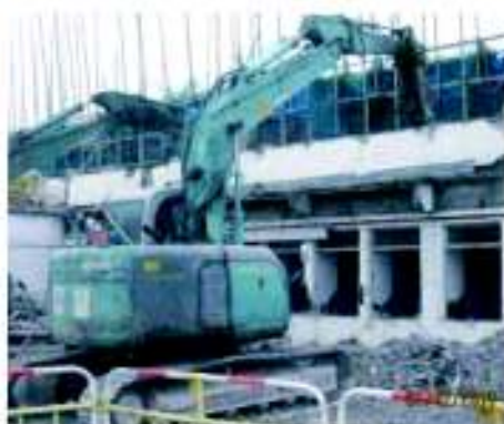
11. Spraying with water during cutting
