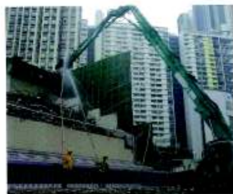
10. Demolishing opposite end bay after removal of props
