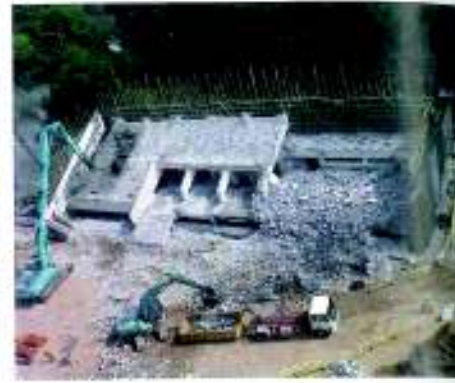
12. Demolishing spectator seating
