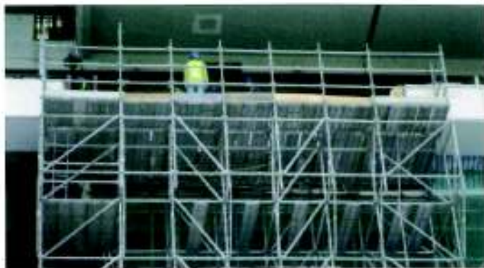
Platform under cantilever structure
