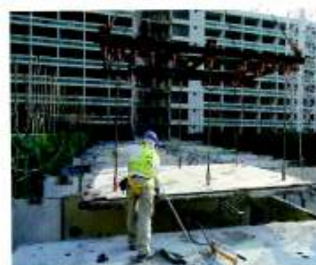
7. Lifting up Precast Slab Panel (1)
