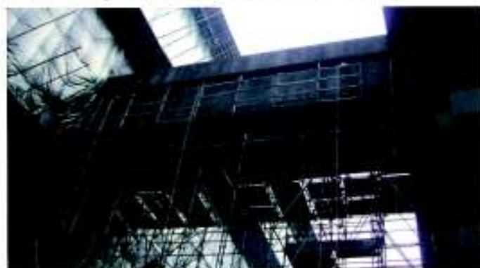
Erecting platform under structure to be demolished
