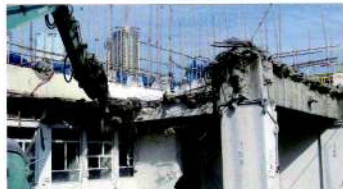
5. Crushing slab behind beam (slab temporarily supported on 3 sides)
