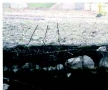
4. Beam breaking completed
