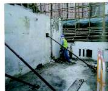
9. Exposing Joints of Precast Wall Panel
