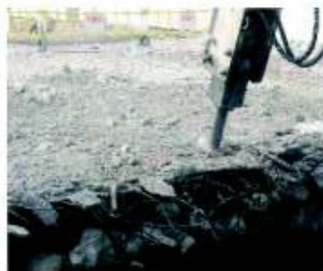
5. Breaking up slab behind beam
