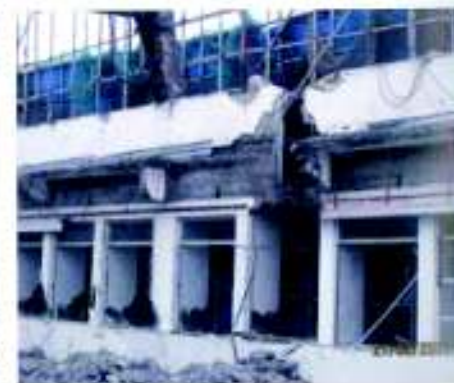
9. Cutting horizontal rebar
