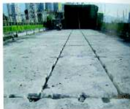
3. Exposing Joints of Precast Slab Panels
