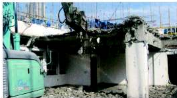
4. Crushing slab behind beam (slab temporarily supported on 3 sides)
