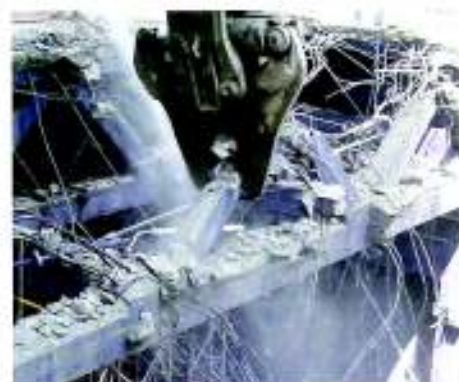
4. Crushing of diagonal chords
