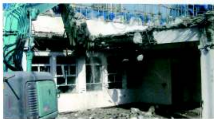
2. Crushing continues on left side of beam
