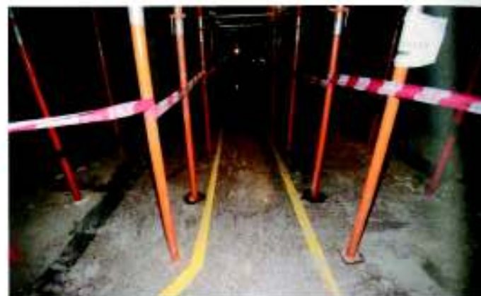
Props with horizontal tubular bracing by couplers
