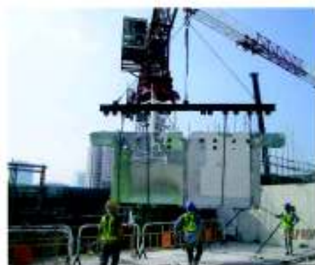
15. Lifting up Precast Wall Panel (2)
