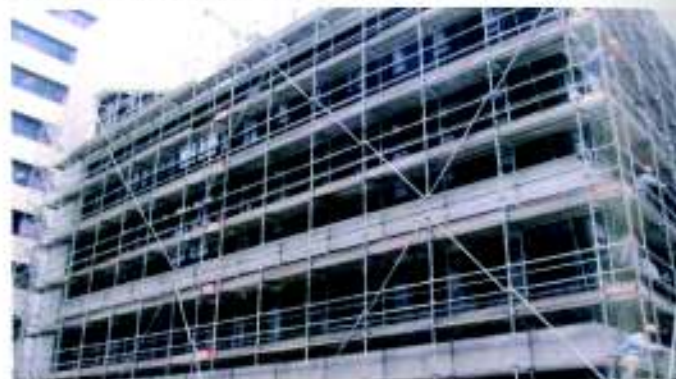
Frame system used as external scaffolding
