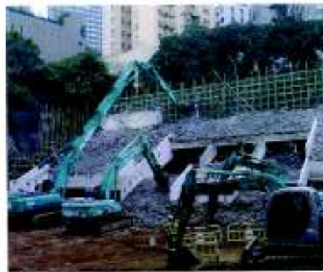
11. Demolishing end column/wall supporting main cantilever girder
