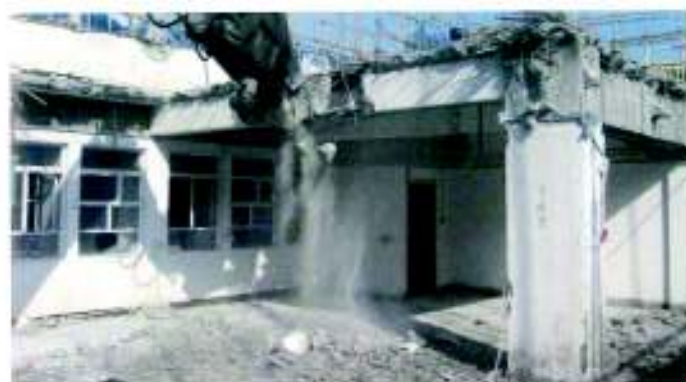
1. Crushing of beam starting at mid span
