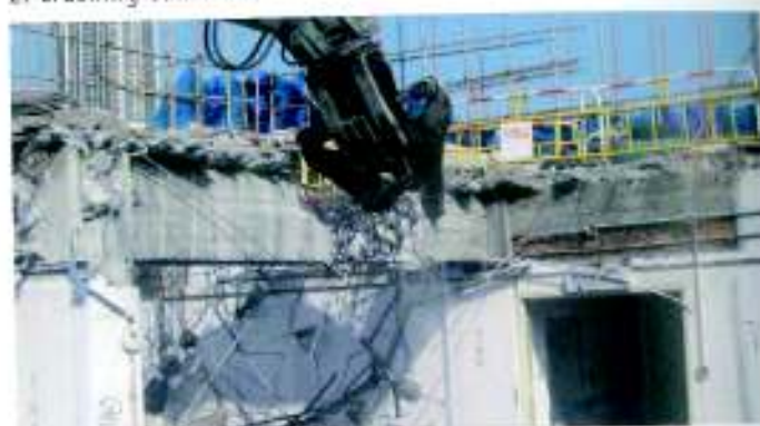
4. Exposing beam rebars
