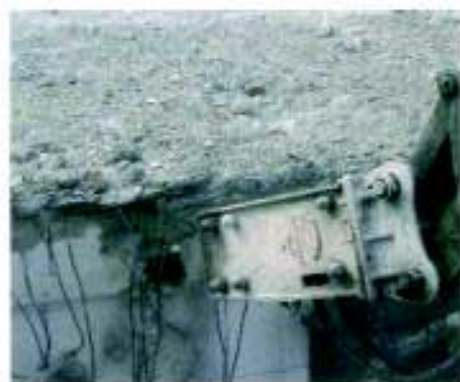
1. Breaking beam at mid-span
