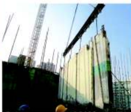
14. Lifting up Precast Wall Panel (1)
