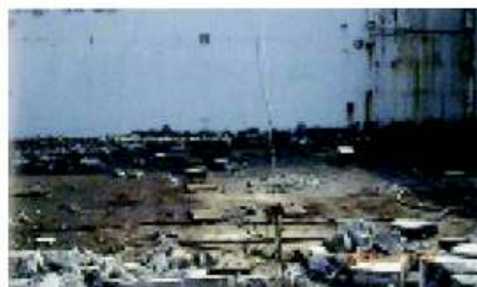
Example 6 Wall Demolition by Manual Method Using Chain and Block
