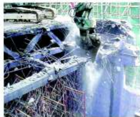
5. Crushing of bottom chords
