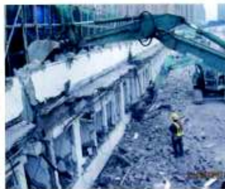
5. Breaking the parapet
