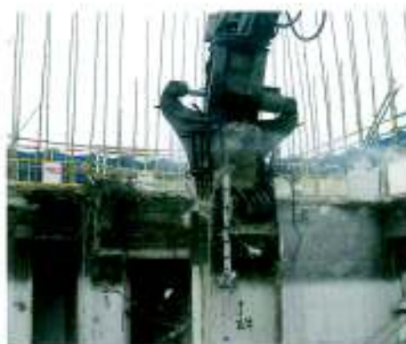
1. Crushing starts with surrounding area vacated
