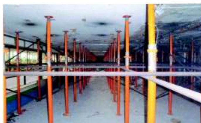
Props with horizontal steel angle bracing by welding
