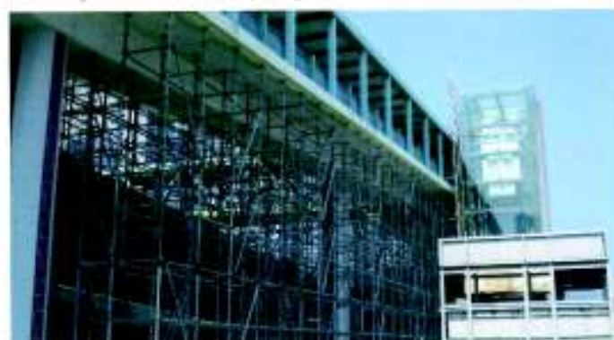
Frame system used as propping for excessive height
