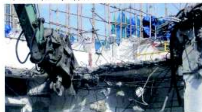
7. Repeating slab panel demolition
