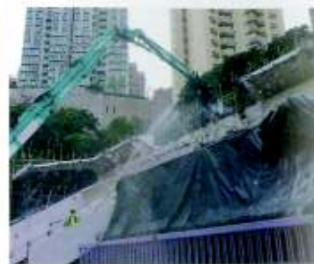
6. Crushing remaining main cantilever girder
