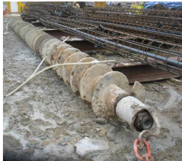
Photo HU5.2 – Auger Drilling Rod
