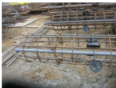
Photo HU5.11 – Prefabricated Steel Cage
