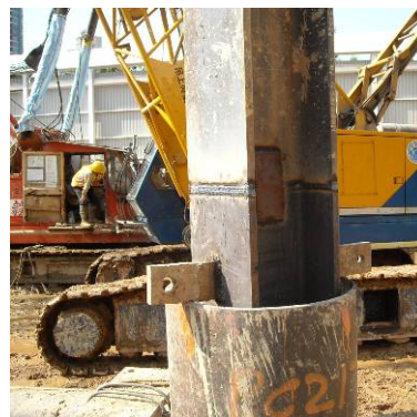
Photo HU3.9 – Splicing of Steel H-pile
