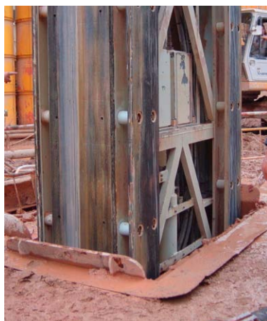
Photo HU6.5 – Excavation by Hydromill within Guide Walls
