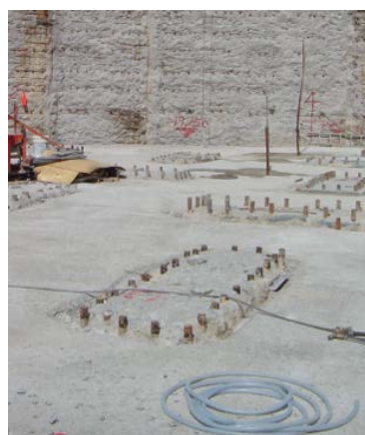
Photo HU6.11 – Finished Barrette after Concreting / Grouting
