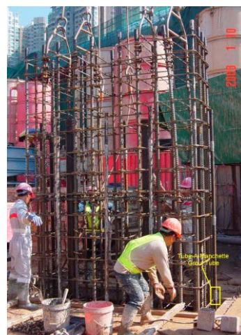
Photo HU6.9 – Lowering Reinforcement Cage into Excavation Trench
