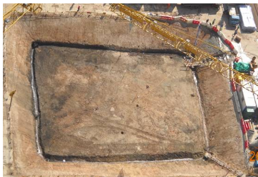
Photo HU7.1 – Open Excavation for Raft Footing Construction
