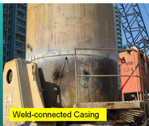
Photo HU2.4 – Extending the Temporary Steel Casing by Bolting or Welding Connections
