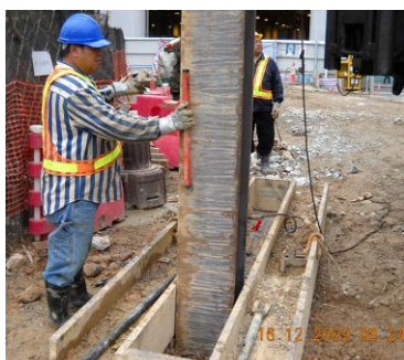
Photo HU1.4 – Checking Verticality
