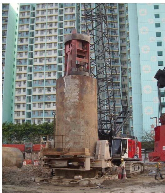
Photo HU2.3 – Excavation using Hammer Grab inside Temporary Steel Casing.
