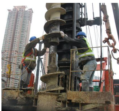
Photo HU5.4 – Extension of Auger Drilling Rod
