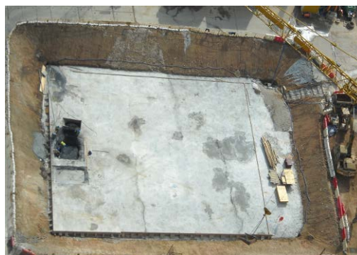
Photo HU7.2 – Blinding the Bottom Level of the Raft Footing
