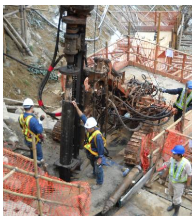
Photo HU4.4 – Checking Alignment of Mini-pile
