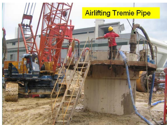
Photo HU2.9 – Cleaning of Pile Base using Airlifting Method by Compressed Air
