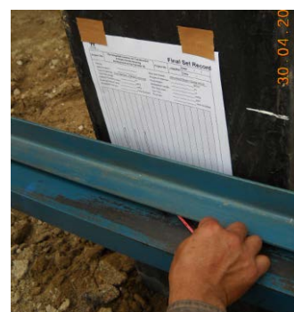
Photo HU1.12 – Close-up of Final Set Measurement
