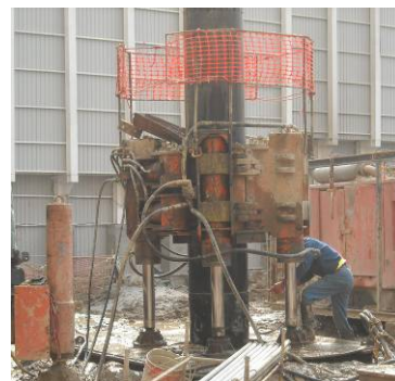
Photo HU3.15 – Extracting Temporary Steel Casing by Hydraulic Jack under Adverse Condition
