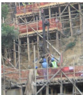
Photo HU4.1 – Drilling Rig for Mini-pile on Working Platform
