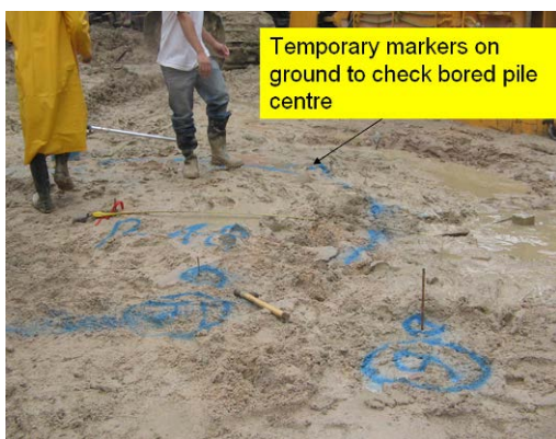
Photo HU2.1 – Setting-Out of Pile on Ground
