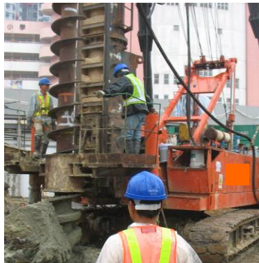
Photo HU5.5 – Drilling Completed to the Required Depth of Pile
