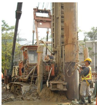
Photo HU3.8 – Splicing of Temporary Casing
