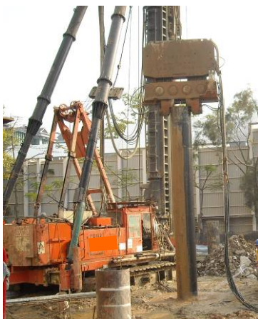
Photo HU3.14 – Extracting Temporary Steel Casing by Vibrating Hammer
