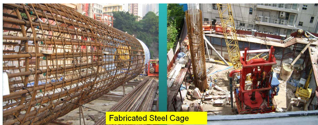
Photo HU2.8 – Installation of Steel Reinforcement Cage inside the Bored Pile Shaft using Crawler Crane
