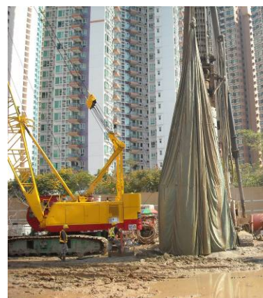
Photo HU3.6 – Double Shelter for Noise and Dust Reduction during Piling
