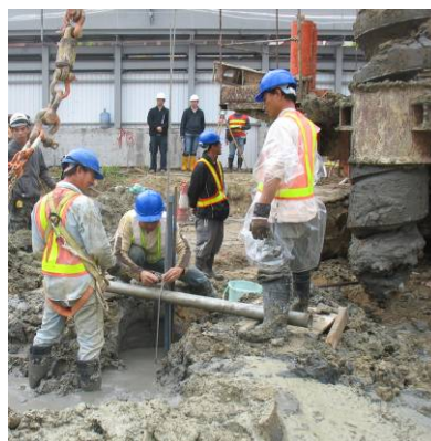
Photo HU5.14 – Stabilizing the Steel Cage (in Grout) by U-bolts
