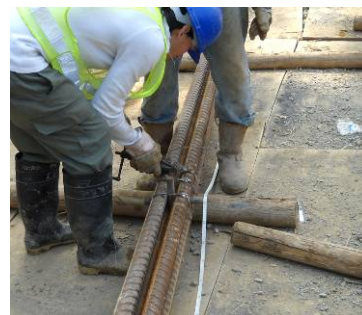
Photo HU4.8 – Prefabrication of Steel Bars
