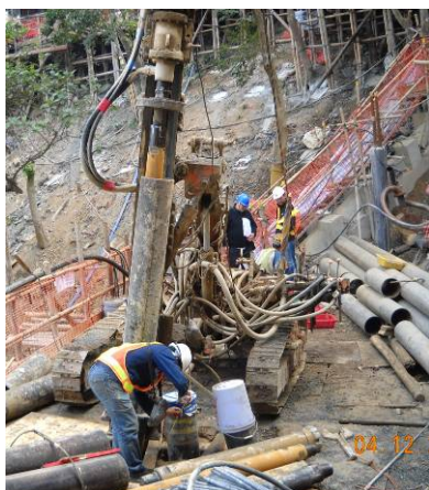
Photo HU4.3 – Drilling Work in Progress (Raking Min-pile)
