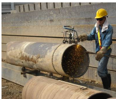
Photo HU3.7 – Casing Joint Preparation
