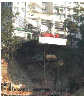
Photo HU4.1 – Drilling Rig for Mini-pile on Working Platform
