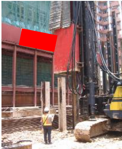
Figure H7.6(b) – Noise Muffler Enclosing Hydraulic Hammer during Percussive Piling Work
