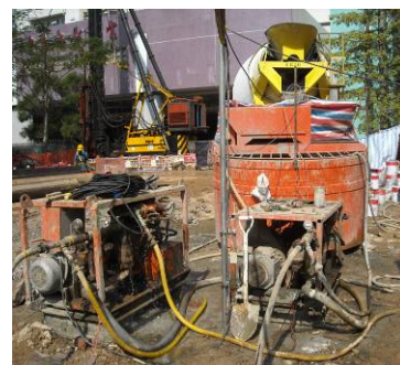
Photo HU3.12 – Air-lifting before Grouting Work
