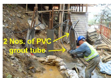
Photo HU4.10 – Completion of Pile by Cement Grouting
