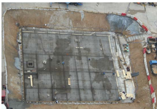
Photo HU7.3 – Reinforcement Fixing for the Bottom Slab
