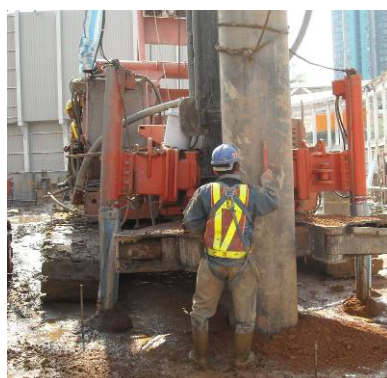
Photo HU3.1 – Drilling with the first Temporary Casing
