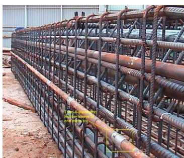
Photo HU6.7 – Reinforcement Cage Pre-fabricated on Site
