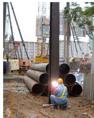
Photo HU1.6 – Connection of Pile by Welding
