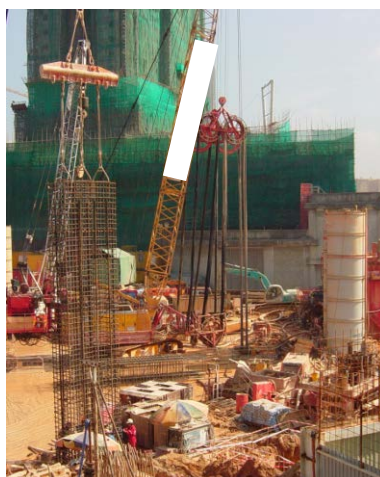
Photo HU6.8 – Lifting Reinforcement Cage
