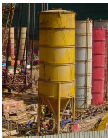
Photo HU6.2 – Silos on Site for Re-circulation of Bentonite Slurry
