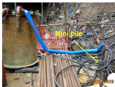
Photo HU4.7 – Air Lifting at Completion of Drilling
