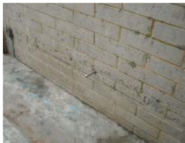
Figure H7.4(b) – Settlement Monitoring Marker on Wall
