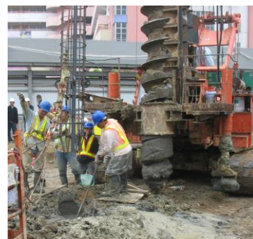
Photo HU5.12 – Installation of Steel Cage into the Pile Shaft
