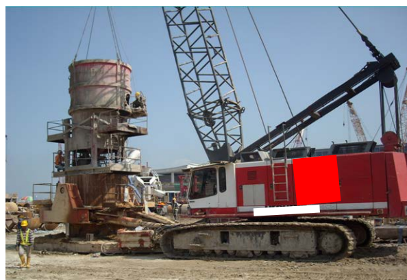
Photo HU2.10 – Placing Tremie Concrete with Gradual Extraction of the Temporary Steel Casing Concurrently
