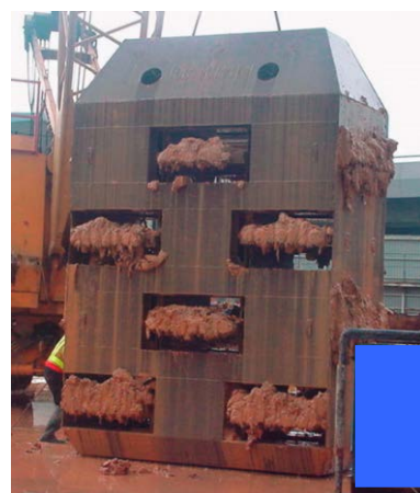
Photo HU6.6 – Scrapers used to Clean Trench sides by Removing Excess Filter Cake
