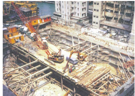
Figure H7.1(b) – Shored Excavation
