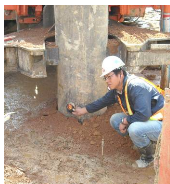
Photo HU3.2 – Checking Alignment
