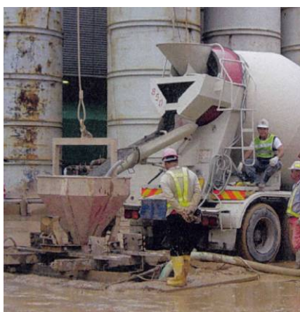
Photo HU6.10 – Tremie Concreting for Barrette
