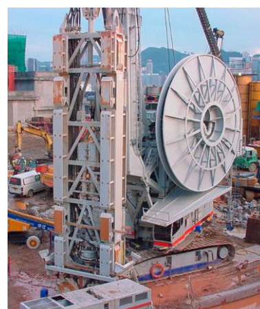
Photo HU6.3 – The Hydromill Machine for Trench Excavation
