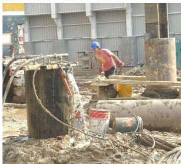
Photo HU3.13 – Cement Grouting for the Socketed H-Pile
