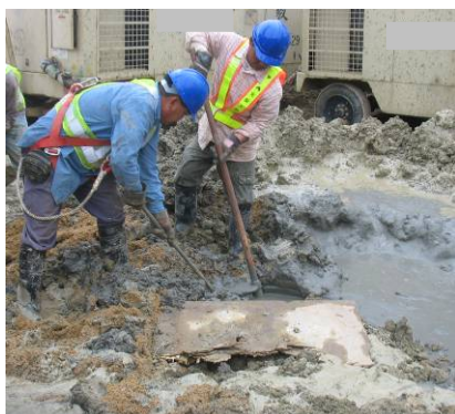
Photo HU5.10 – Completion of Grouting Work
