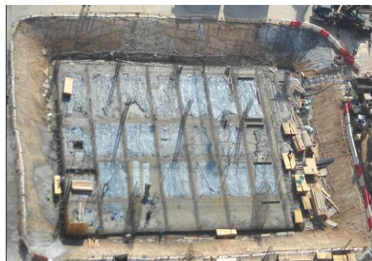
Photo HU7.4 – Concreting for the Bottom Slab
