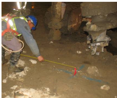
Photo HU5.1 – Setting Out of Pile
