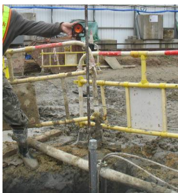
Photo HU5.13 – Surveying of the Top Level of Steel Bar
