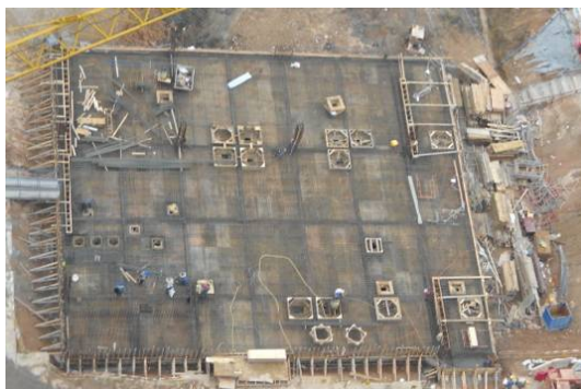
Photo HU7.7 – Formwork Erection and Reinforcement Fixing for the Top Slab
