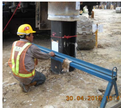
Photo HU1.11 – Final Set Measurement
