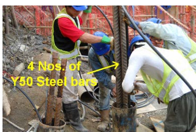
Photo HU4.9 – Installation of Steel Bars
