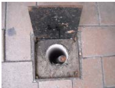
Figure H7.4(a) – Settlement Monitoring Marker on Ground
