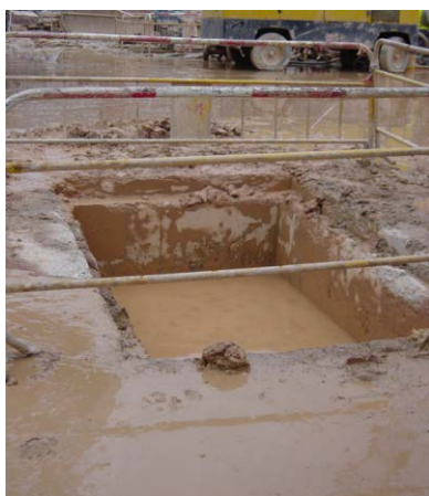
Photo HU6.1 – Shallow Trench formed and surrounded by Guide Walls and filled by Bentonite Slurry
