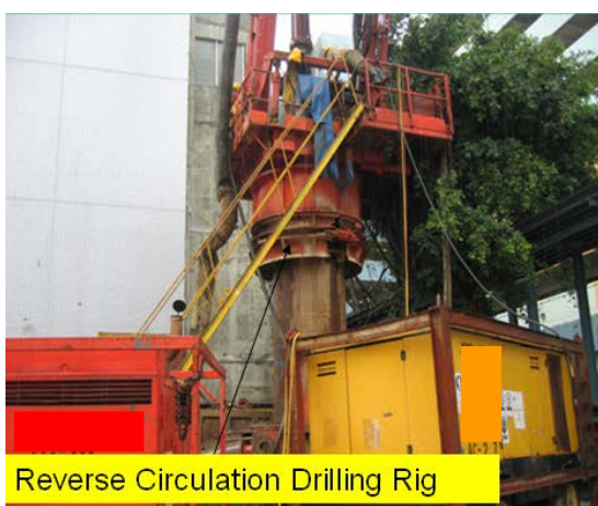
Photo HU2.5 – Excavation of rock or similar hard material using Reverse Circulation Drilling Rig for Formation of the Rock Socket.
