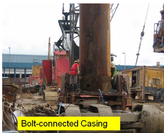
Photo HU2.4 – Extending the Temporary Steel Casing by Bolting or Welding Connections
