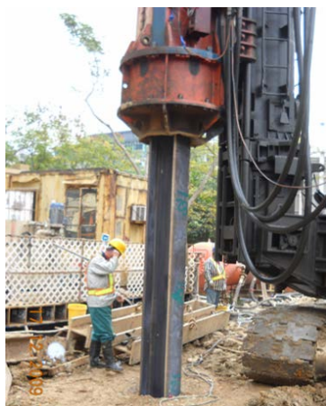
Photo HU1.8 – Pitching to the Required Depth
