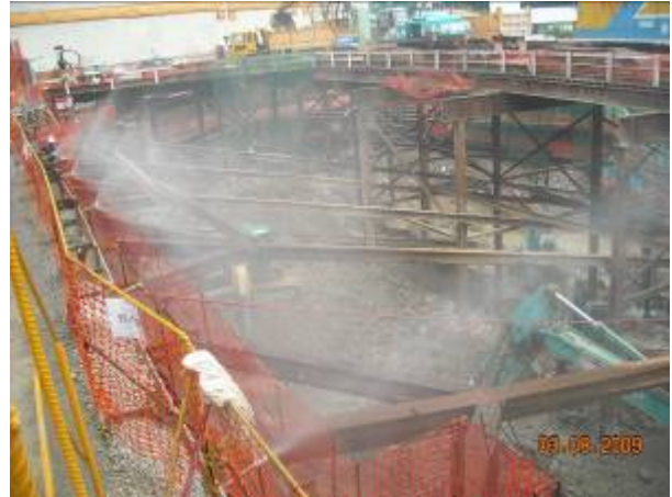
Figure H7.8 – Spraying of Water for Dust Suppression
