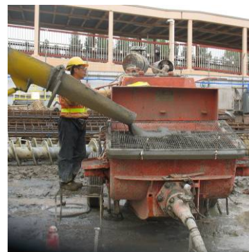
Photo HU5.6 – Grouting Work of Pile
