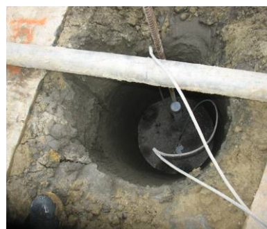
Photo HU5.15 – Inspection of Grout at Top Level of Pile before Backfill
