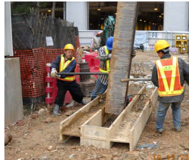
Photo HU1.3 – Installation of Pile in Correct Position
