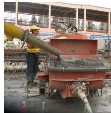
Photo HR5.6 – Grouting Work of Pile
