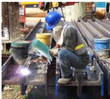
Photo HR1.1 – Welding of Pile Shoes
