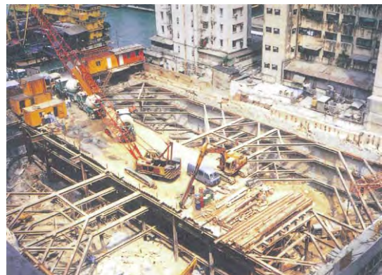
Figure H7.1(b) – Shored Excavation
