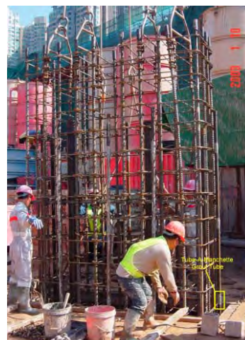
Photo HR6.9 – Lowering Reinforcement Cage into Excavation Trench
