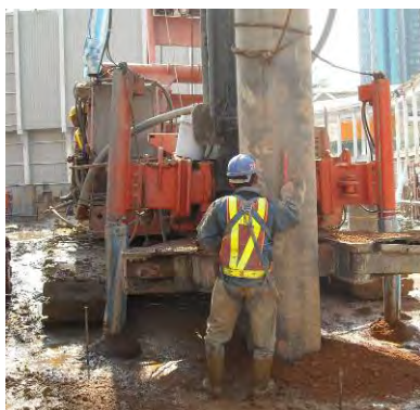
Photo HR3.1 – Drilling with the first Temporary Casing
