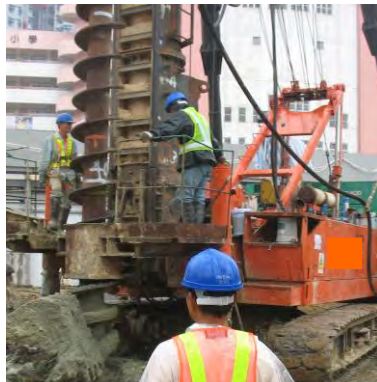
Photo HR5.5 – Drilling Completed to the Required Depth of Pile
