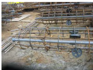
Photo HR5.11 – Prefabricated Steel Cage
