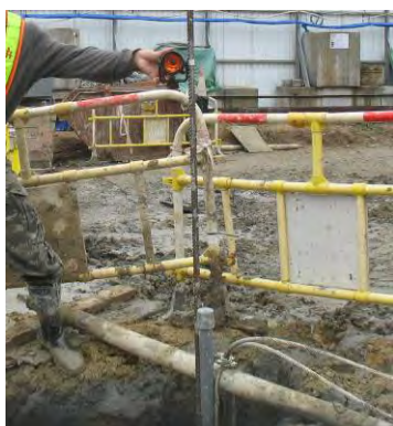
Photo HR5.13 – Surveying of the Top Level of Steel Bar
