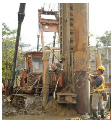
Photo HR3.8 – Splicing of Temporary Casing
