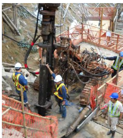
Photo HR4.4 – Checking Alignment of Mini-pile
