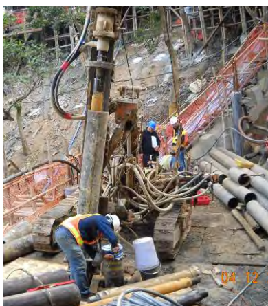
Photo HR4.3 – Drilling Work in Progress (Raking Min-pile)
