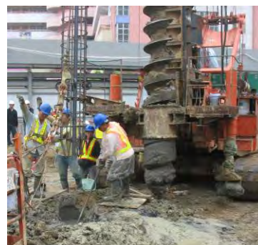
Photo HR5.12 – Installation of Steel Cage into the Pile Shaft
