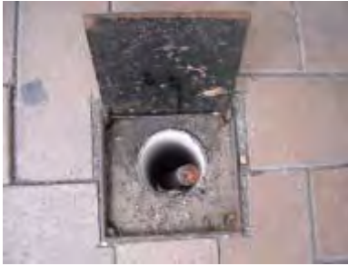
Figure H7.4.1 – Settlement Monitoring Marker on Ground
