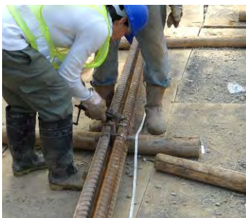
Photo HR4.8 – Prefabrication of Steel Bars
