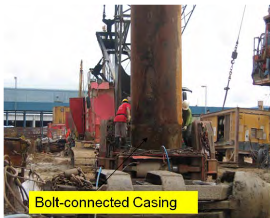
Photo HR2.4 – Extending the Temporary Steel Casing by Bolting or Welding Connections
