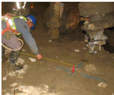
Photo HR5.1 – Setting Out of Pile
