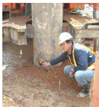
Photo HR3.2 – Checking Alignment
