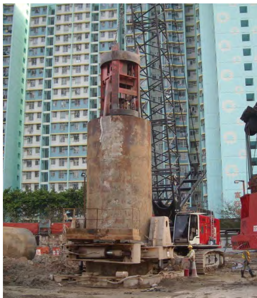
Photo HR2.3 – Excavation using Hammer Grab inside Temporary Steel Casing.
