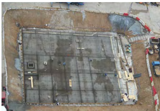
Photo HR7.3 – Reinforcement Fixing for the Bottom Slab
