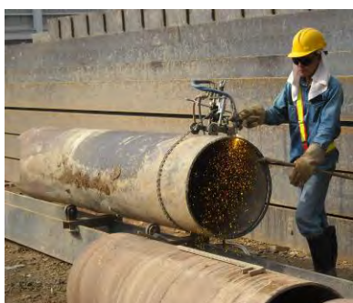
Photo HR3.7 – Casing Joint Preparation
