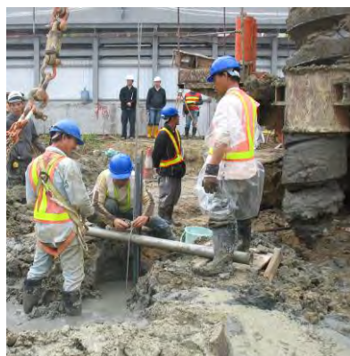
Photo HR5.14 – Stabilizing the Steel Cage (in Grout) by U-bolts
