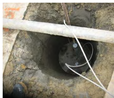
Photo HR5.15 – Inspection of Grout at Top Level of Pile before Backfill
