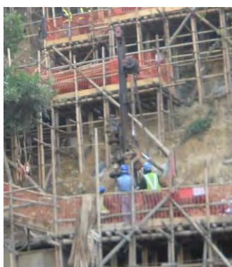
Photo HR4.1 – Drilling Rig for Mini-pile on Working Platform
