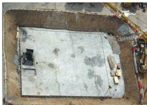
Photo HR7.2 – Blinding the Bottom Level of the Raft Footing
