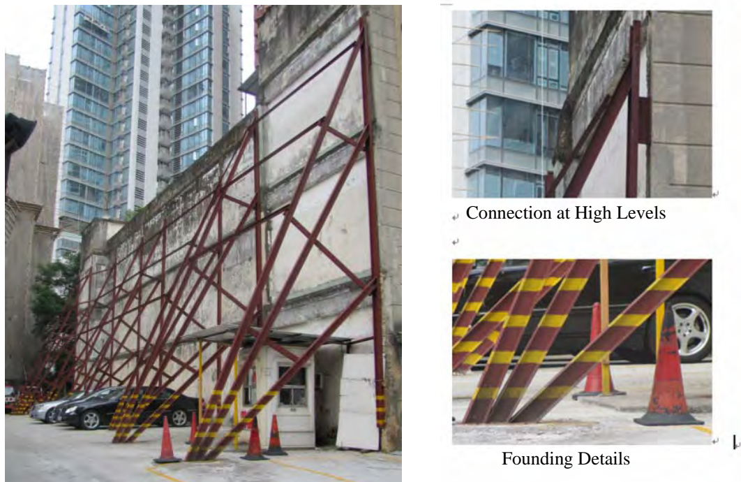
Figure H7.3 – Double Raking Shore to Enhance Stability of Building
