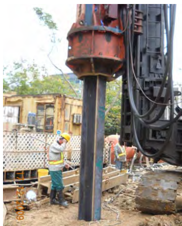
Photo HR1.8 – Pitching to the Required Depth
