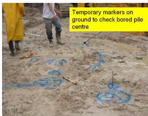
Photo HR2.1 – Setting-Out of Pile on Ground
