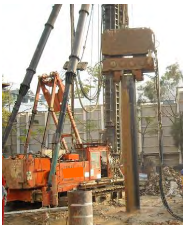
Photo HR3.14 – Extracting Temporary Steel Casing by Vibrating Hammer
