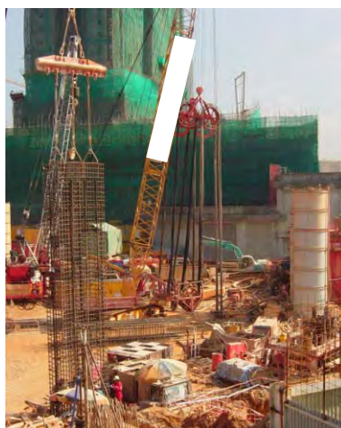
Photo HR6.8 – Lifting Reinforcement Cage
