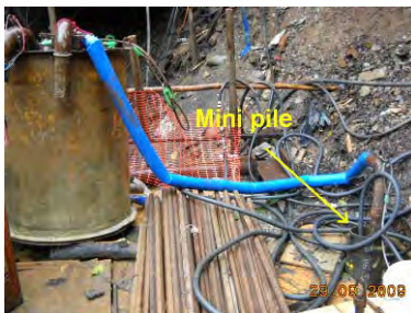
Photo HR4.7 – Air Lifting at Completion of Drilling
