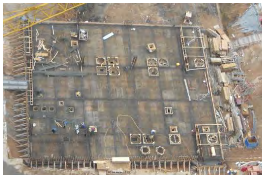
Photo HR7.7 – Formwork Erection and Reinforcement Fixing for the Top Slab
