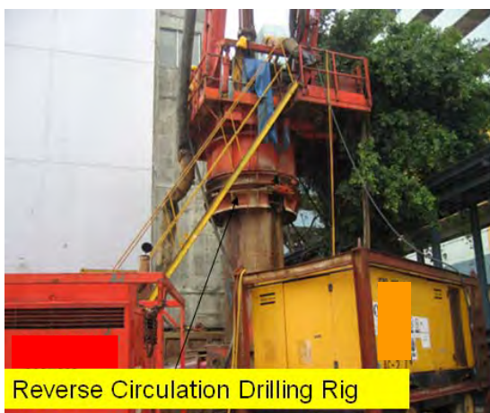
Photo HR2.5 – Excavation of rock or similar hard material using Reverse Circulation Drilling Rig for Formation of the Rock Socket.
