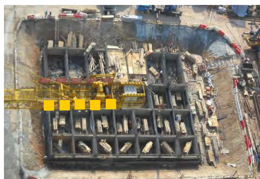
Photo HR7.6 – concreting for the Walls
