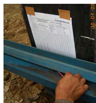
Photo HR1.11(b) – Close-up of Final Set Measurement
