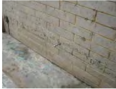
Figure H7.4.2 – Settlement Monitoring Marker on Wall
