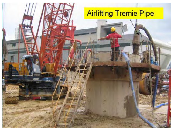
Photo HR2.9 – Cleaning of Pile Base using Airlifting Method by Compressed Air
