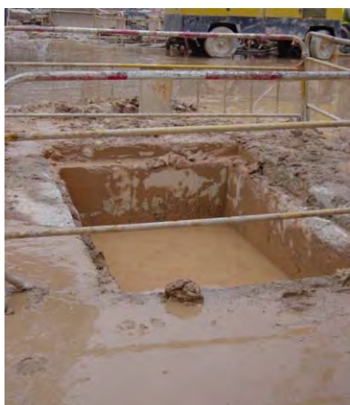
Photo HR6.1 – Shallow Trench formed and surrounded by Guide Walls and filled by Bentonite Slurry
