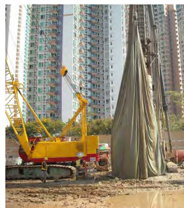
Photo HR3.6 – Double Shelter for Noise and Dust Reduction during Piling
