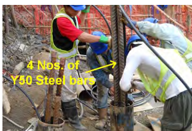
Photo HR4.9 – Installation of Steel Bars
