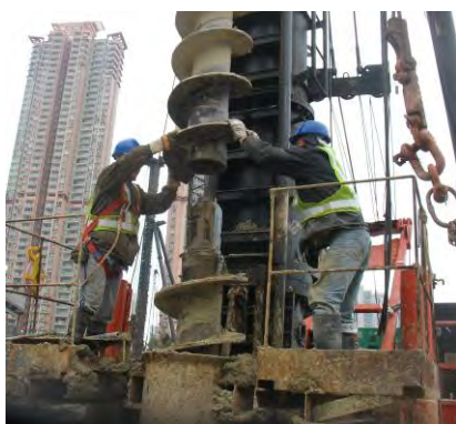
Photo HR5.4 – Extension of Auger Drilling Rod
