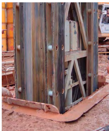
Photo HR6.5 – Excavation by Hydromill within Guide Walls
