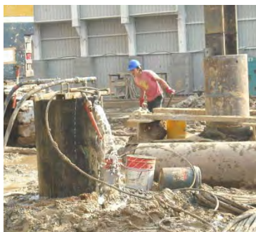
Photo HR3.13 – Cement Grouting for the Socketed H-Pile
