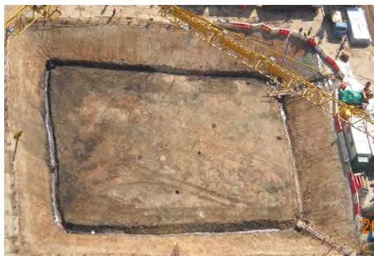
Photo HR7.1 – Open Excavation for Raft Footing Construction
