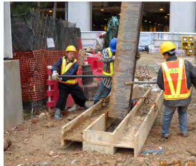
Photo HR1.3 – Installation of Pile in Correct Position
