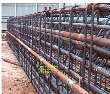
Photo HR6.7 – Reinforcement Cage Pre-fabricated on Site
