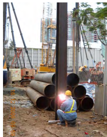
Photo HR1.6 – Connection of Pile by Welding
