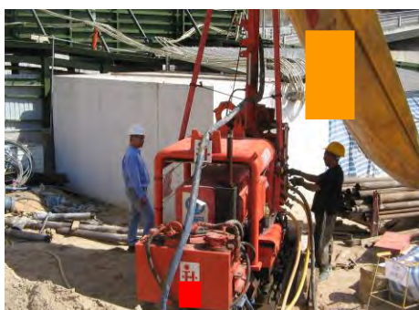
Photo HR2.11 – Rotary Drilling Rig for Concrete Core Test
