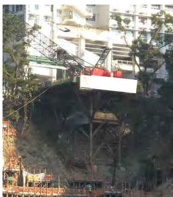
Photo HR4.1 – Drilling Rig for Mini-pile on Working Platform
