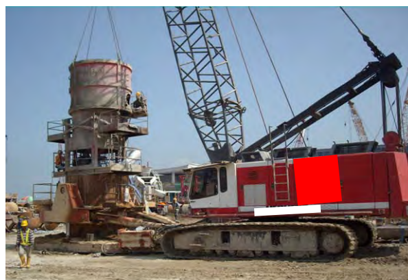
Photo HR2.10 – Placing Tremie Concrete with Gradual Extraction of the Temporary Steel Casing Concurrently
