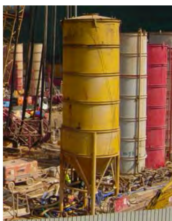
Photo HR6.2 – Silos on Site for Re-circulation of Bentonite Slurry
