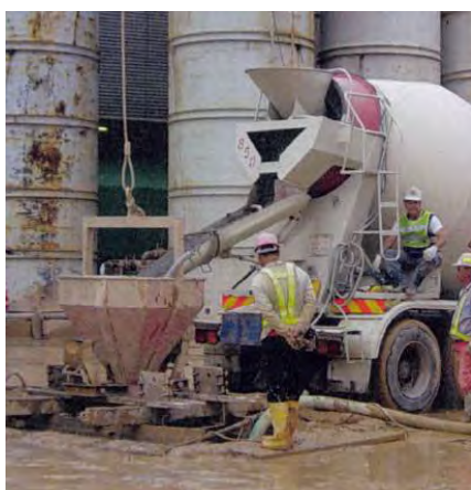
Photo HR6.10 – Tremie Concreting for Barrette
