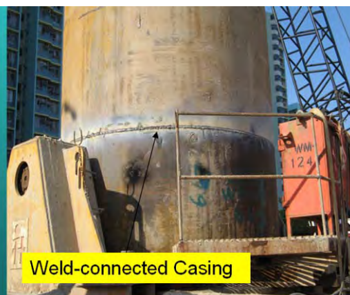
Photo HR2.4 – Extending the Temporary Steel Casing by Bolting or Welding Connections
