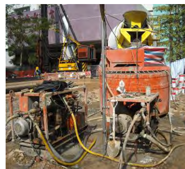
Photo HR3.12 – Air-lifting before Grouting Work
