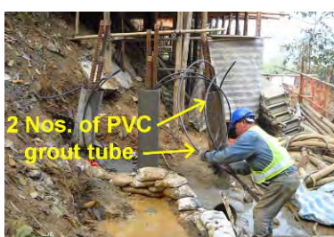
Photo HR4.10 – Completion of Pile by Cement Grouting
