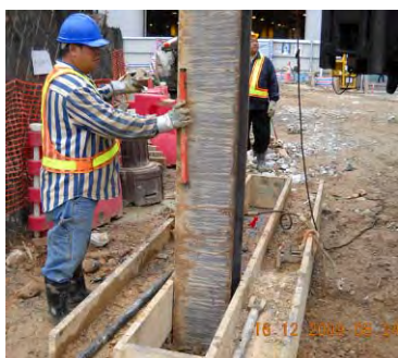
Photo HR1.4 – Checking Verticality
