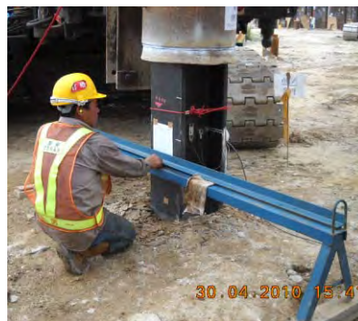
Photo HR1.11(a) – Final Set Measurement
